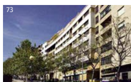
73. Apartment Building, Granada avenue, Javier Campos López. 74. Apartment Building, Alcantarilla District, Eduardo Duro Almazán.
