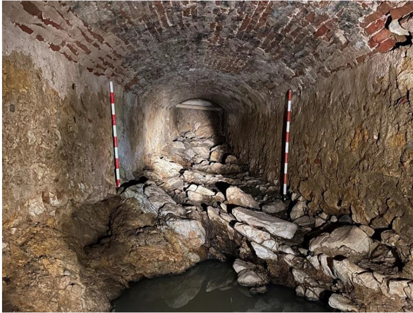
Fig. 3. Interior del colector
