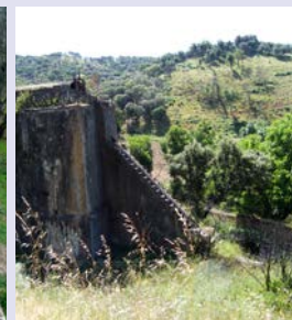
[145] Hydroelectric mill in Rivera del Huéznar
