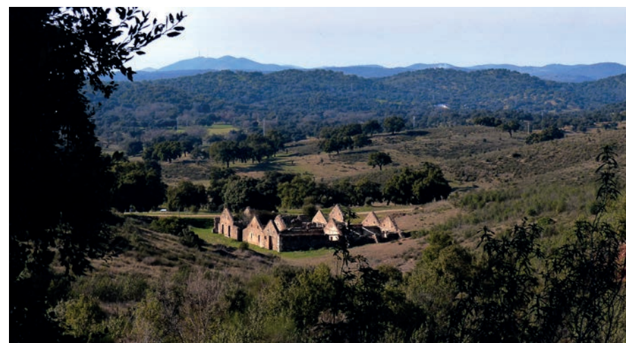
[255] Panoramic view of mining facilities ruins
