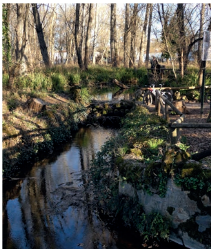
[247] Drainage canal of the pool
