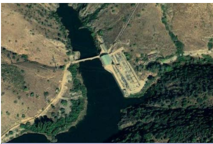
[148] Location of the power plant of El Pintado
