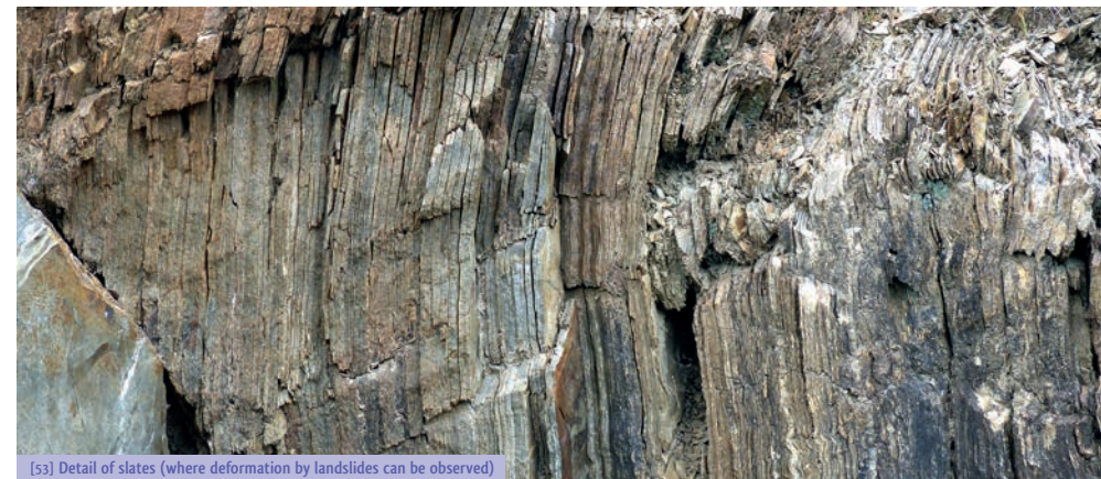
[53] Detail of slates (where deformation by landslides can be observed)
