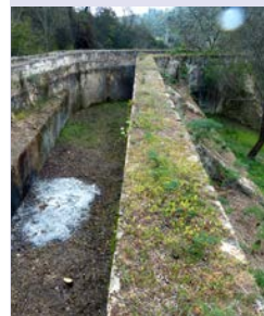
[144] Canal (water pipe) of a hydraulic mill
