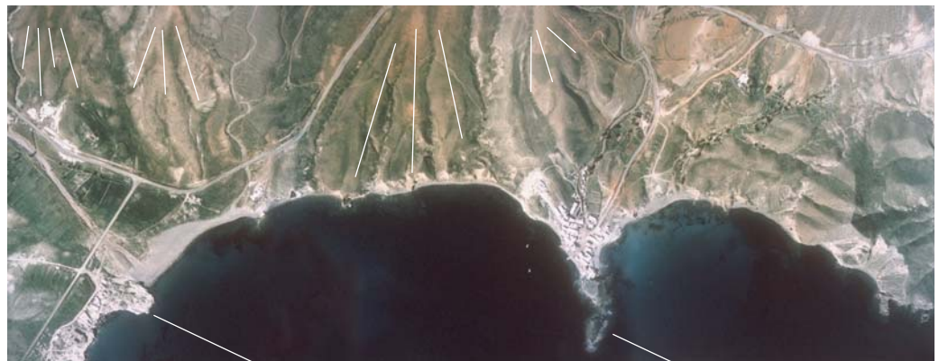
Aerial view of La Isleta-Los Escullos in which phase 2 alluvial fans may be observed, with a schematic overlay.
