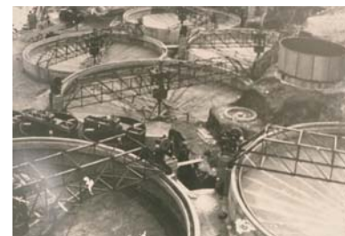
System of cleaning tanks in operation (Photo, Evaristo Gil Picón).
