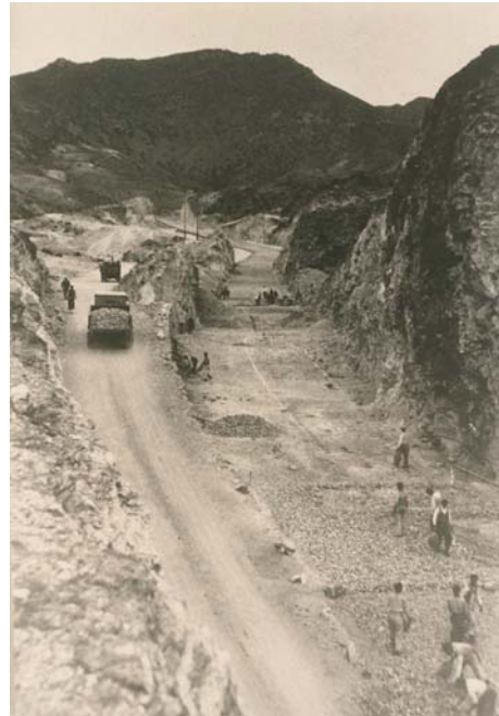
Opening of the track that connected the Cerro del Cinto mine workings with the grading and concentration plant. This infrastructure already meant an enormous advance that opened up the possibility of mechanising the quarrying system (Photo, Evaristo Gil Picón).
