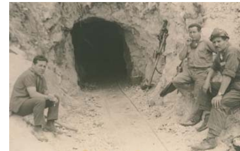
Mine entrance of 'Lode 340' during the period of maximum activity in the mining district of Rodalquilar. The photograph is taken roughly in the 50's decade (Photo, Evaristo Gil Picón).
