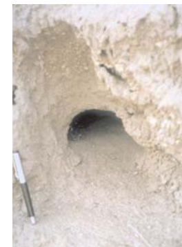
Drainage pipe close to local base level.
