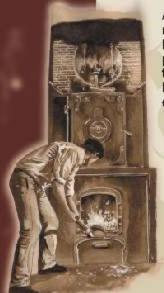
Although resin has been used since ancient times to make pitch with which to waterproof roofs and boats, its industrial use and the distillation of turpentine or pine resin started in the 18th century. The process treats the resin via distillation, passing through various boilers named large, autoclave and decanter in order to eliminate all types of impurities.
