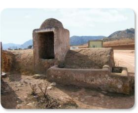
After the first kilometre we encounter a large cistern and a trough [2], once constructions of great strategic value in such an arid landscape. The underground cistern has a rectangular floor and barrel vault ceiling. Behind it we find the rainwater decanter that feeds it.
