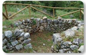
Limekilns were furnaces where limestone was turned into whitewash. The raw materials were plentiful in these mountains, as was the gorse that was used as fuel. The average limekiln needed over three thousand to fire.
