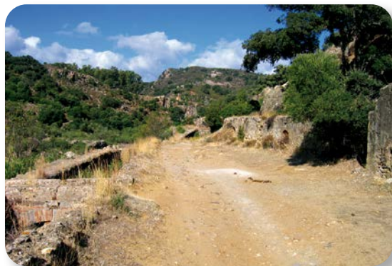
The Royal Artillery Factory was built during the second half of the 18th century for the manufacture of war material (mainly bombs) necessary for the defence of the overseas colonies. Numerous munitions were shipped from here to the mouth of the River Palmones during the Great Siege of Gibraltar (1779-1783).
