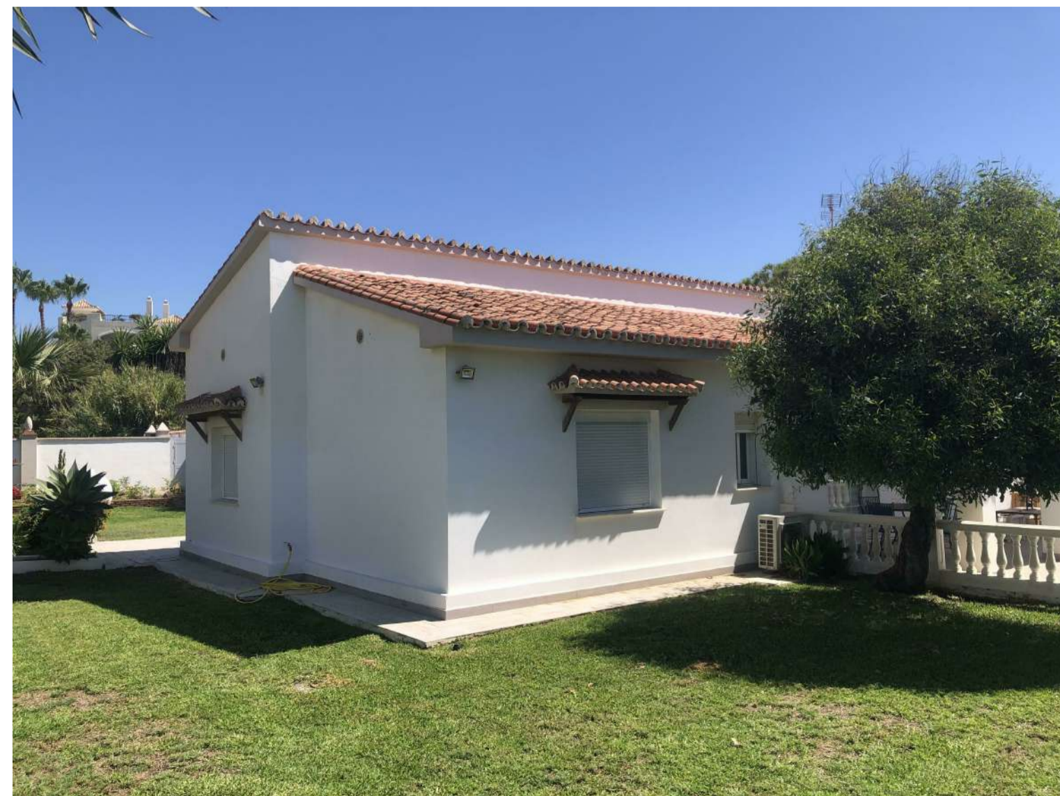
Chalé a demoler (01)
