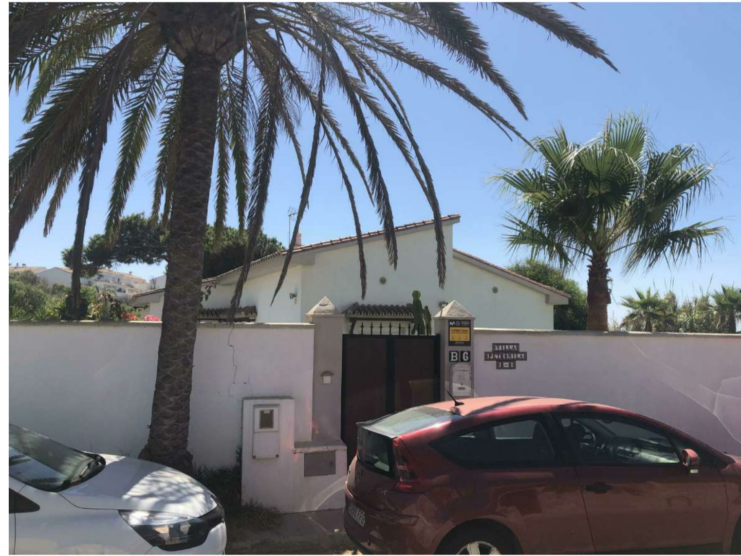
Chalé a demoler (01)
