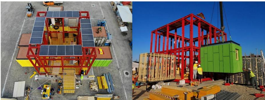
Fig. 7 Prototype in the Solar Village during the assembly phase (Stenzendre, Hungary)
